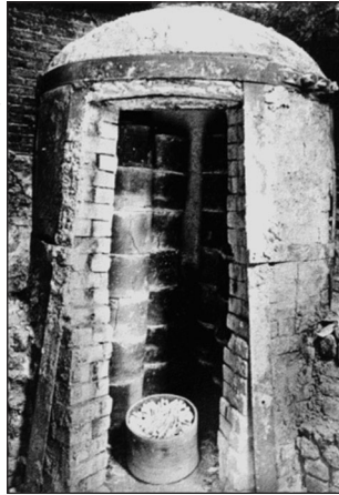
Pl 11 Clay pipe kiln of John Hamilton, Bathurst Court, Belfast, 1912 (after Deane 1914).
